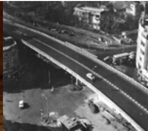
Concrete Hinge as Bearing in Bridge First application in 1965
