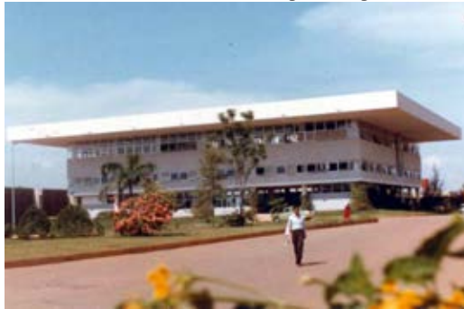
L&T – Office Building, Bangalore
