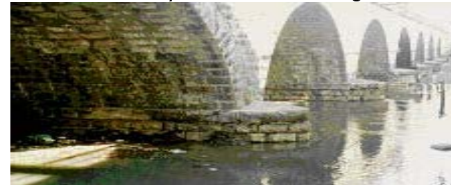
2001 Structural Condition Survey & Repairs
