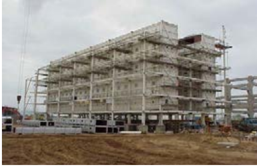
Petronas - Primary Reformer, Malaysia
