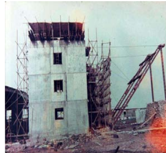
First large panel system of prefabrication in India used for upper 24 floors after thorough full scale load testing - 1973
