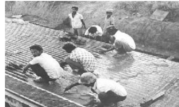
Factory building from Precast North light Girders, Hyper shells, Wall Panels with Beer bottle finish
