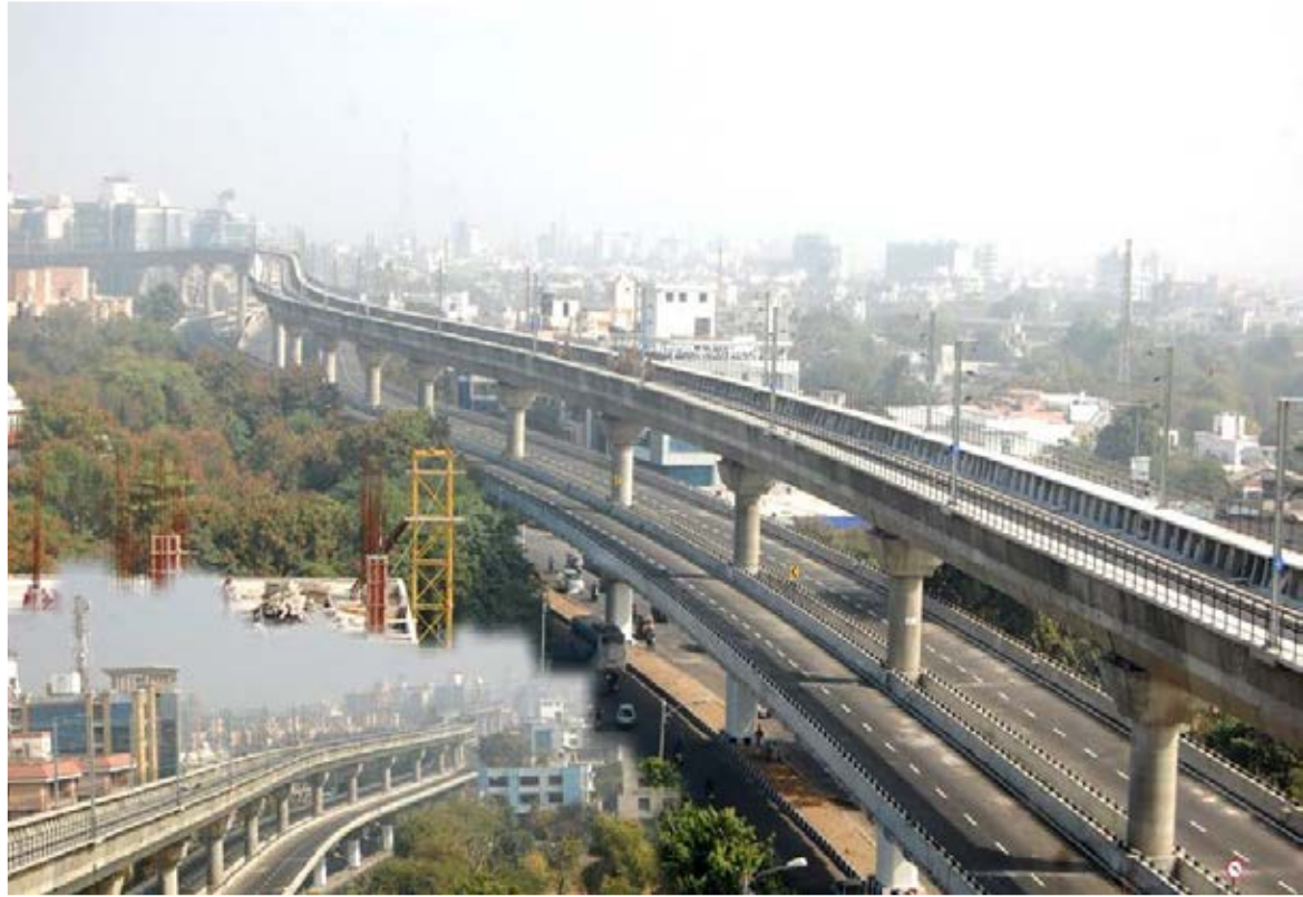
Segmental construction for Four lane flyover with Elevated Metro viaduct supported on a single central pier
