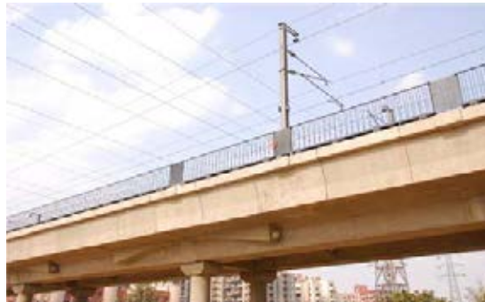
Full Span Precast Deck made integral with Piers
