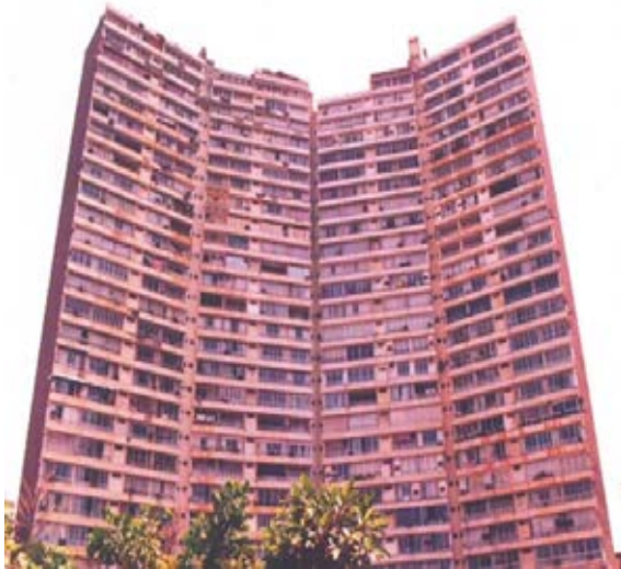
First large panel system of prefabrication in India used for upper 24 floors after thorough full scale load testing - 1973
