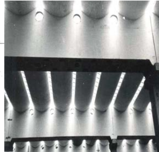
Strip Skylights cheaper than North light & provide brighter light
