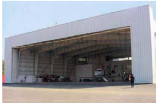
TAJ Air - Hangar, Mumbai
