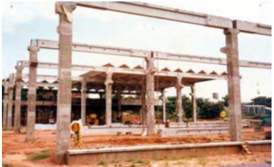
Factory building from Precast Folded Plates, Roof beams, Columns, Wall panels with Beer bottle finish
