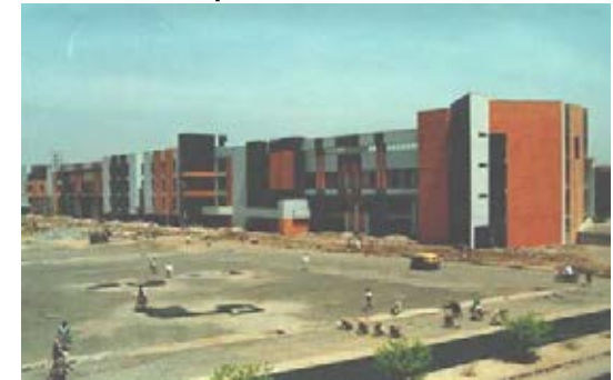
CIDCO –Sanpada Station, Navi Mumbai
