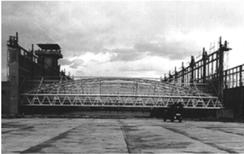
Complete assembly of 90m x 45m roof & lifting vertically by jacks (no use of cranes) - 1981
