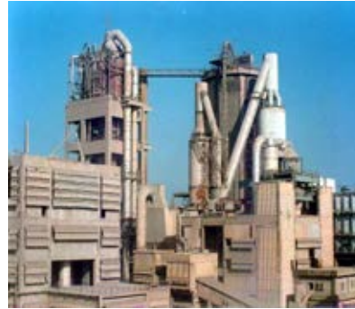
L&T – Cement Plant Upgradation, Awarpur
