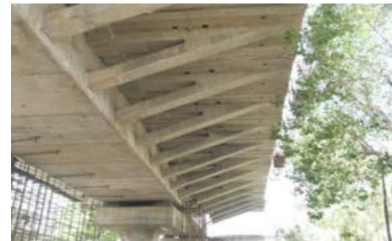
Segmental construction for Four lane flyover with Elevated Metro viaduct supported on a single central pier
