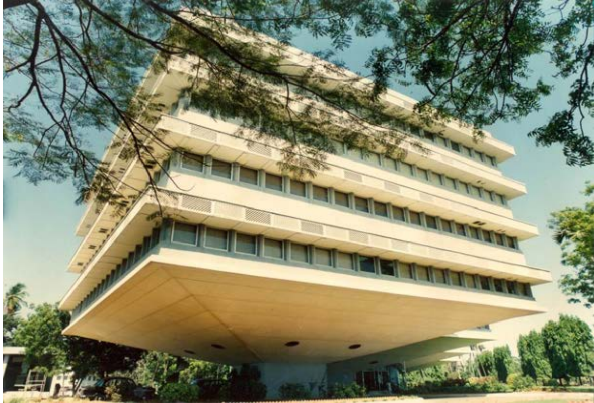
L&T – ECC Administrative Building, Chennai
