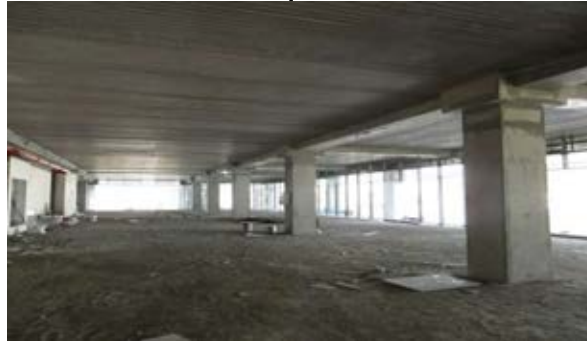
Towers using Precast Beams and Hollow Core Slabs
