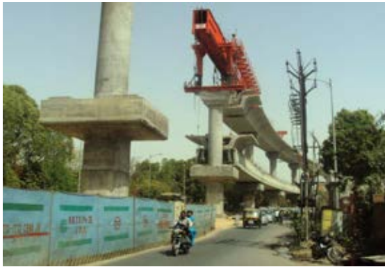
Segmental construction for Four lane flyover with Elevated Metro viaduct supported on a single central pier
