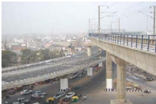
Segmental construction for Four lane flyover with Elevated Metro viaduct supported on a single central pier
