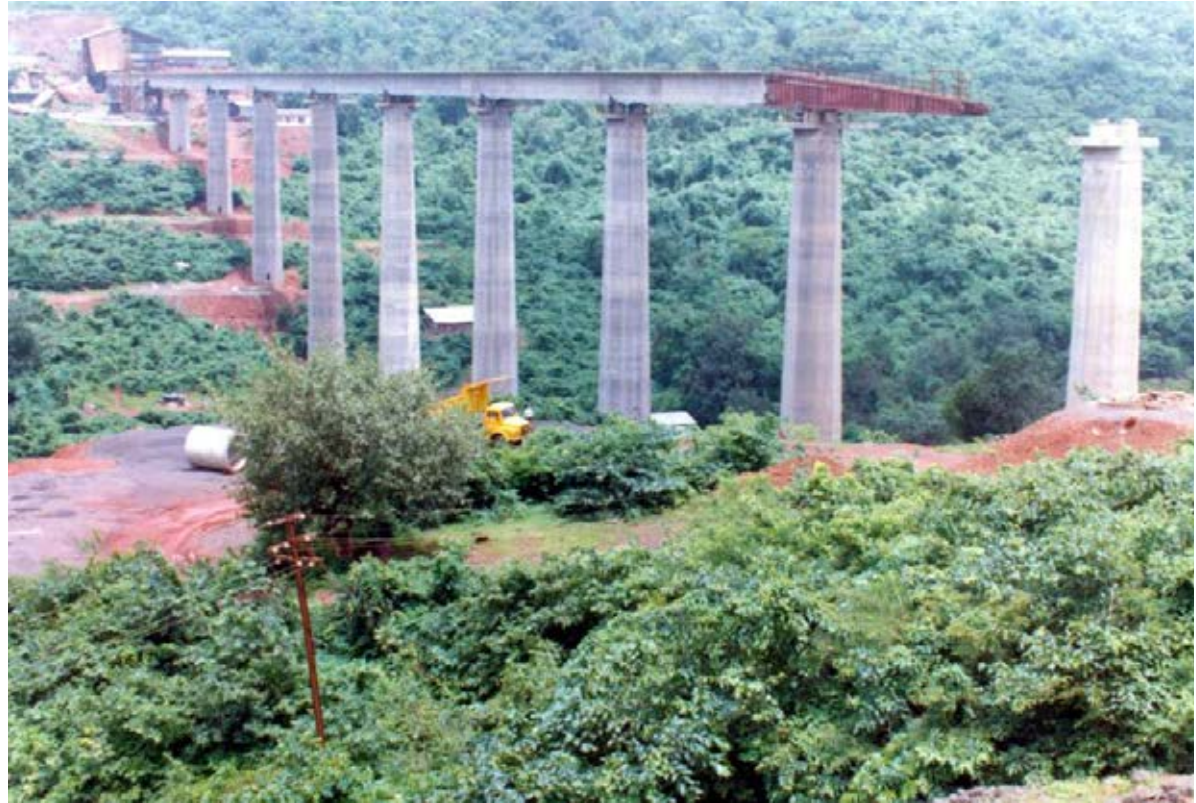
Tallest Pier 62m height, Bridge deck launched by Incremental method (1 st time in India ) for 424m long Viaduct
