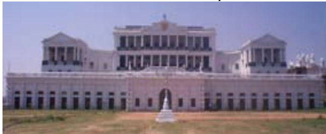
2002 Structural Condition Survey
