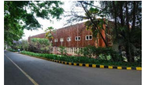
Factory building from Precast Folded Plates, Roof beams, Columns, Wall panels with Beer bottle finish
