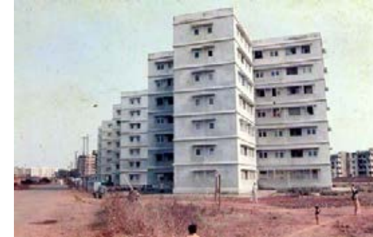
Andheri Precast Mass Housing, Mumbai
