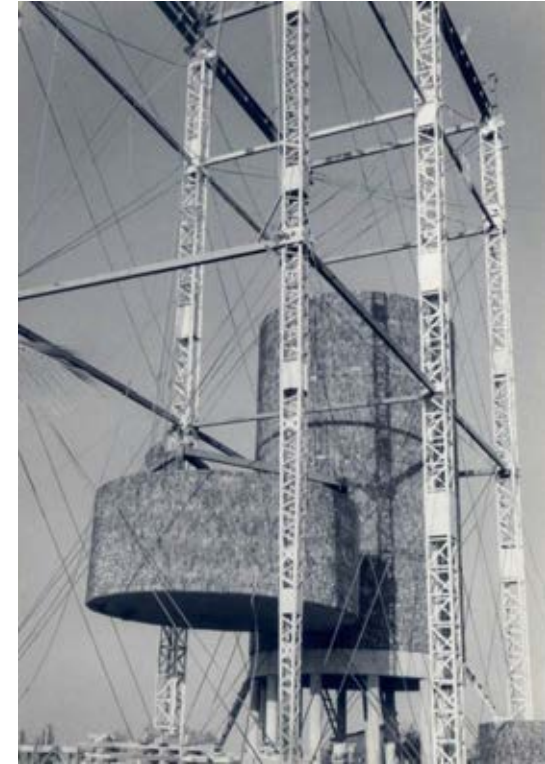
6 Nos Precast Tanks stacked one above
