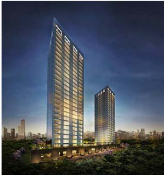
Panchshil – Trump Tower, Pune
