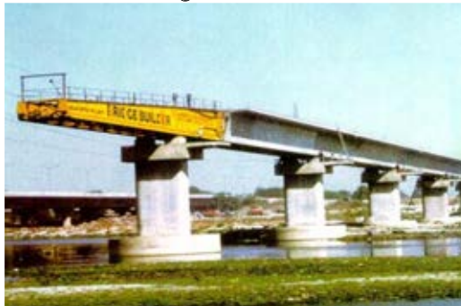
DMRC–Metro Bridge on Yamuna, New Delhi
