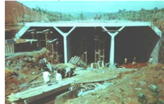
1994 Railway Culvert with 17m overburden
