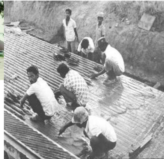
Precast concrete wall Panels with Beer bottle finished surface
