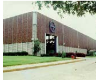
14.5m High Single piece wall panel Largest in India in 1976
