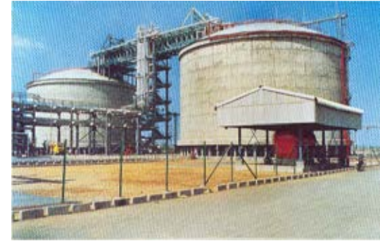
RIL – Ethylene Terminal, Hazira
