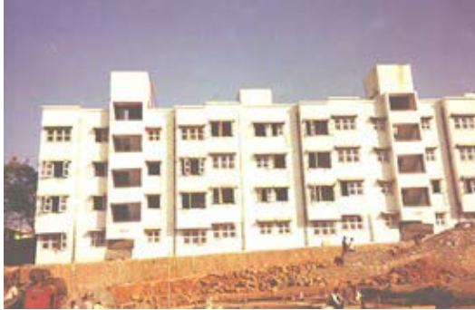
NNP – Dindoshi Mass Housing, Mumbai
