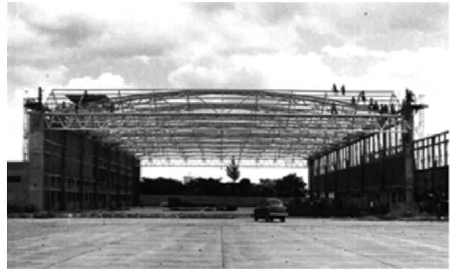
Complete assembly of 90m x 45m roof & lifting vertically by jacks (no use of cranes) - 1981
