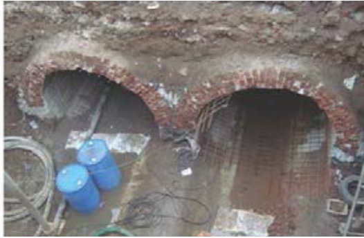
2012 Repairs of Storm Water Mains
