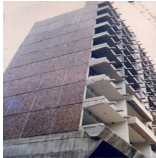
First large panel system of prefabrication in India used for upper 24 floors after thorough full scale load testing - 1973
