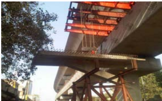
Segmental construction for Four lane flyover with Elevated Metro viaduct supported on a single central pier
