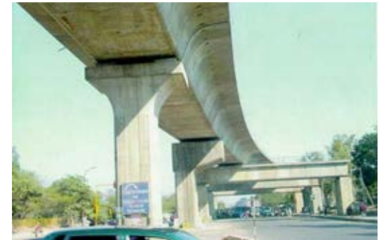
DMRC - Elevated Viaduct, New Delhi
