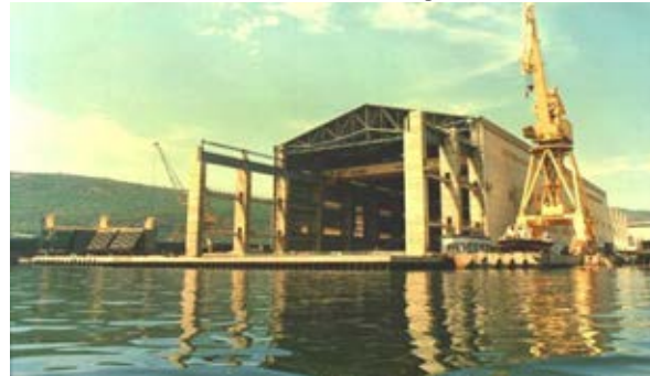
Covered area of shed 18,800m 2
