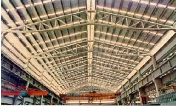
Factory building from all Precast elements like Columns, Gantry Girders, Trusses, Purlins
