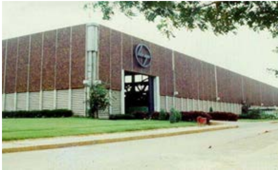
Factory building from Precast North light Girders, Hyper shells, Wall Panels with Beer bottle finish
