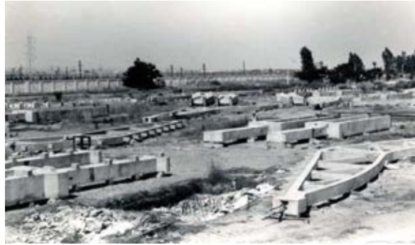
Factory building from all Precast elements like Columns, Gantry Girders, Trusses, Purlins
